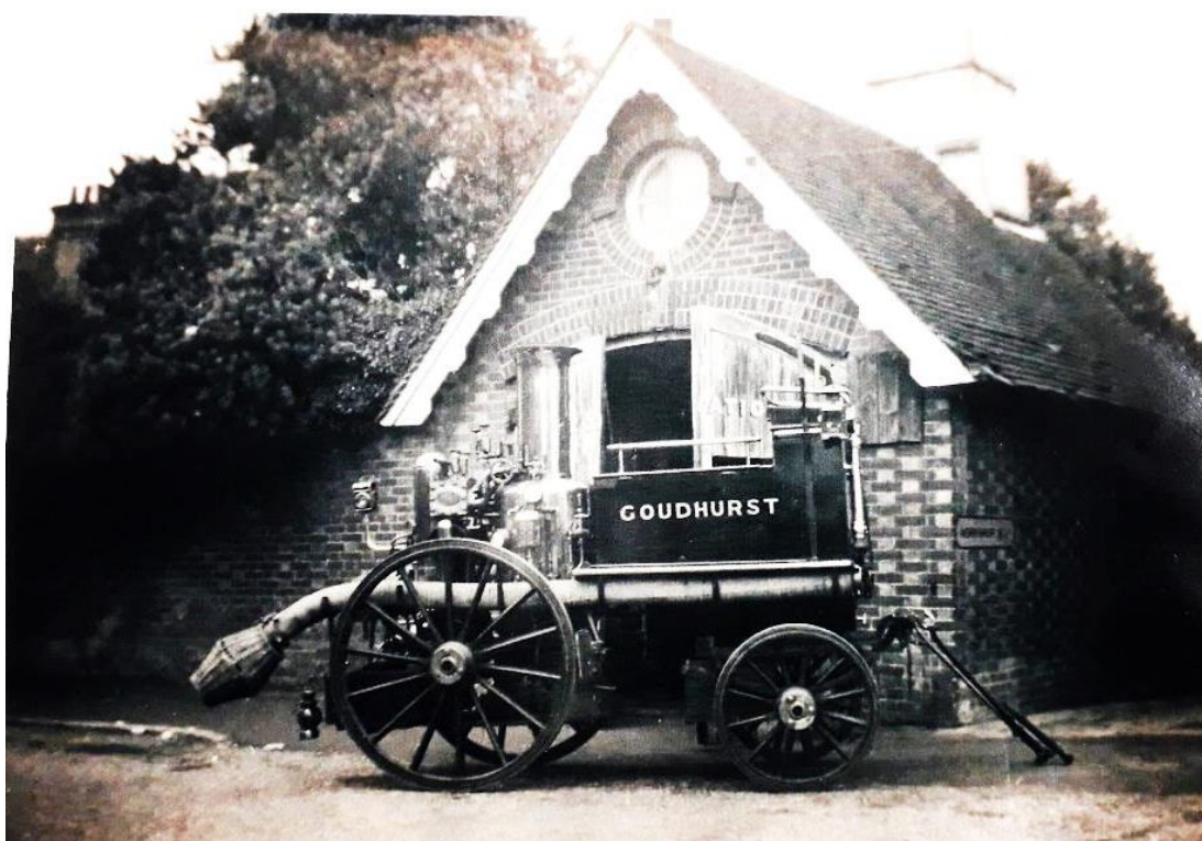
The Shand=Mason Steamer fire engine outside the Old Fire Station in 1930
