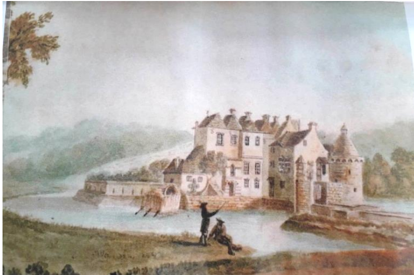
The Old Castle before demolition
